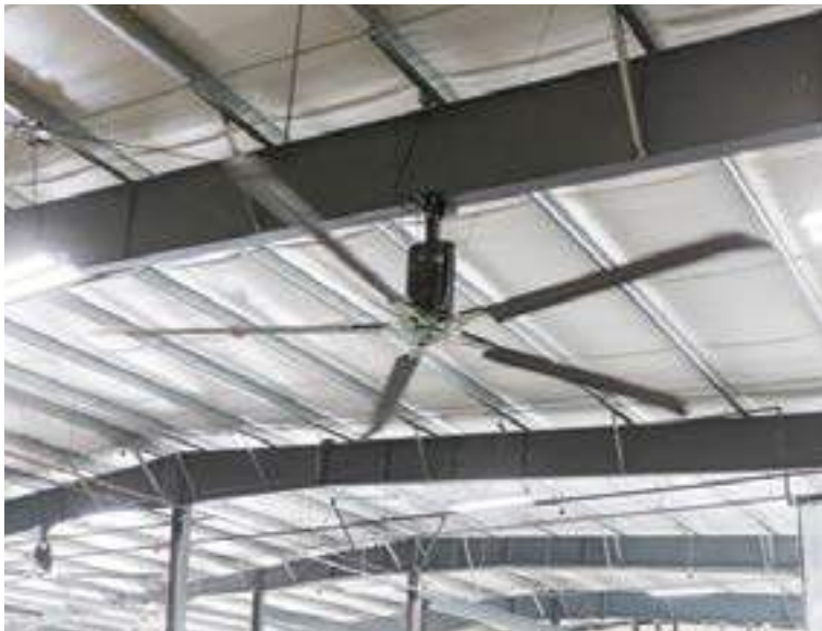
MegaStream HVLS High Volume Low Speed fans like the MegaStream are ideal for providing near ground effect air movement. The unit's low speed operation means it is energy efficient and very quiet.
