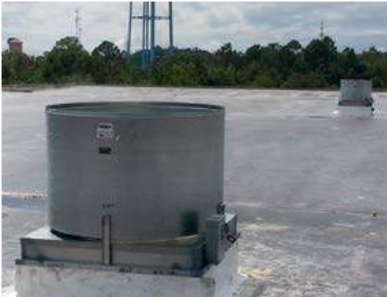
UpStream Fans UpBlast low-silhouette axial fans are designed for exhausting building air to provide general ventilation to hot, stagnant areas. Ideal for individual workspaces.
