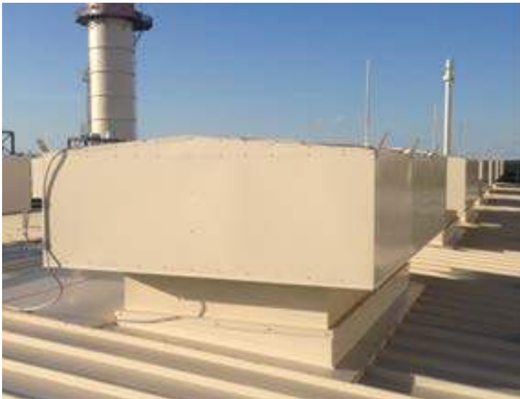
Econovent Econovent ventilators are used for natural air intake or exhaust. The low-profile silhouette looks good on any roof top. It is available in stainless steel, galvanized steel, or aluminum.
