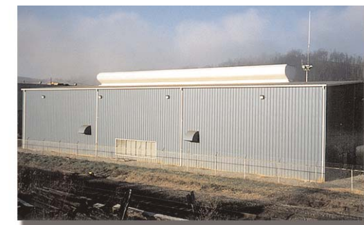
Iron Foundry Building
