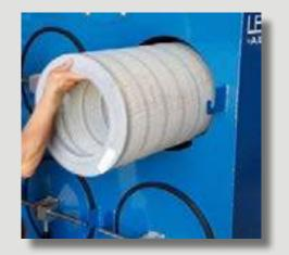
The simple and secure design is widely considered as the best in the industry. Using stainless steel brackets, cross rod and a cast aluminum handle, it will stand up to the toughest environments, both outside and inside your facility. There are no knobs to turn, no moving rails, no interior yokes or threads to catch, or holes to center up — just drop in the door and clamp down. Lift the handle and you're holding the best door the industry has ever seen.
